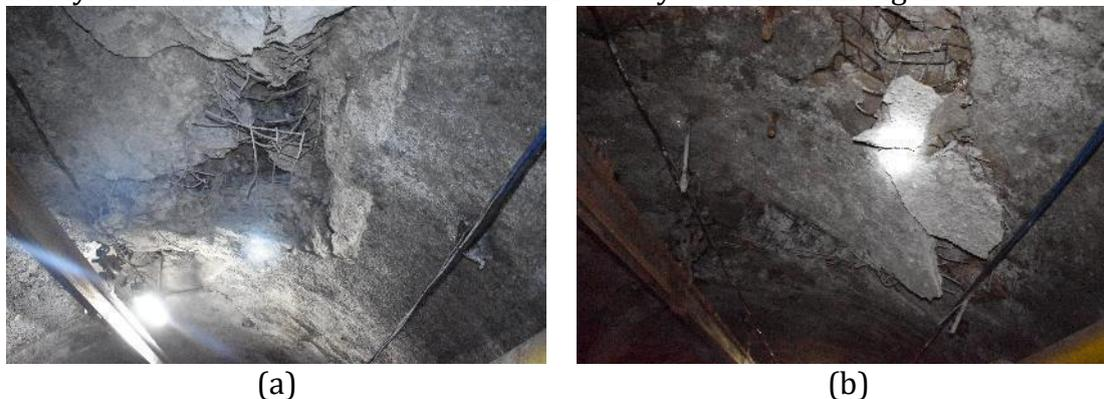
Fig. 2 Failure characteristics of west wing transport roadway
