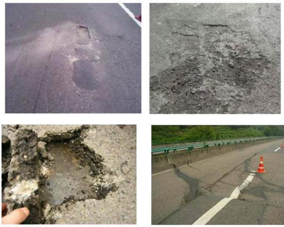
Fig.1 Water damage representative form of pit slot
